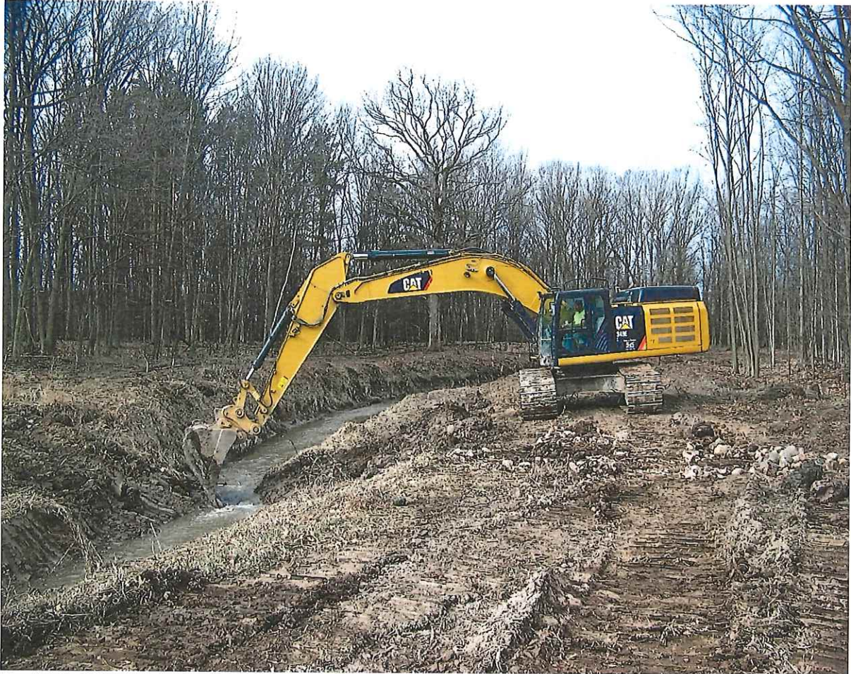
Hoppler Creek Drain Project
